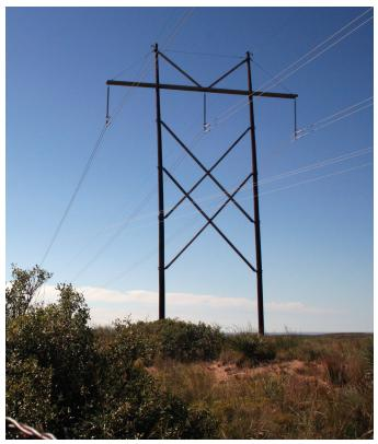
This is a representative 345 kV H-frame transmission line structure that will be used on the Rush Creek project. The structures are typically 100 to 130 feet tall with a 150 foot right-of-way.
