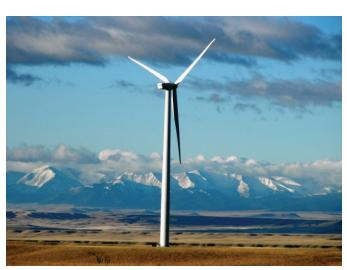
The Rush Creek project is expected to include 300 wind turbines. Each of the wind turbines will have an estimated capacity of 2 megawatts for a 600 megawatt total capacity. The turbine hub height is typically about 260 feet with the tip of the blade being approximately 440 feet tall.
